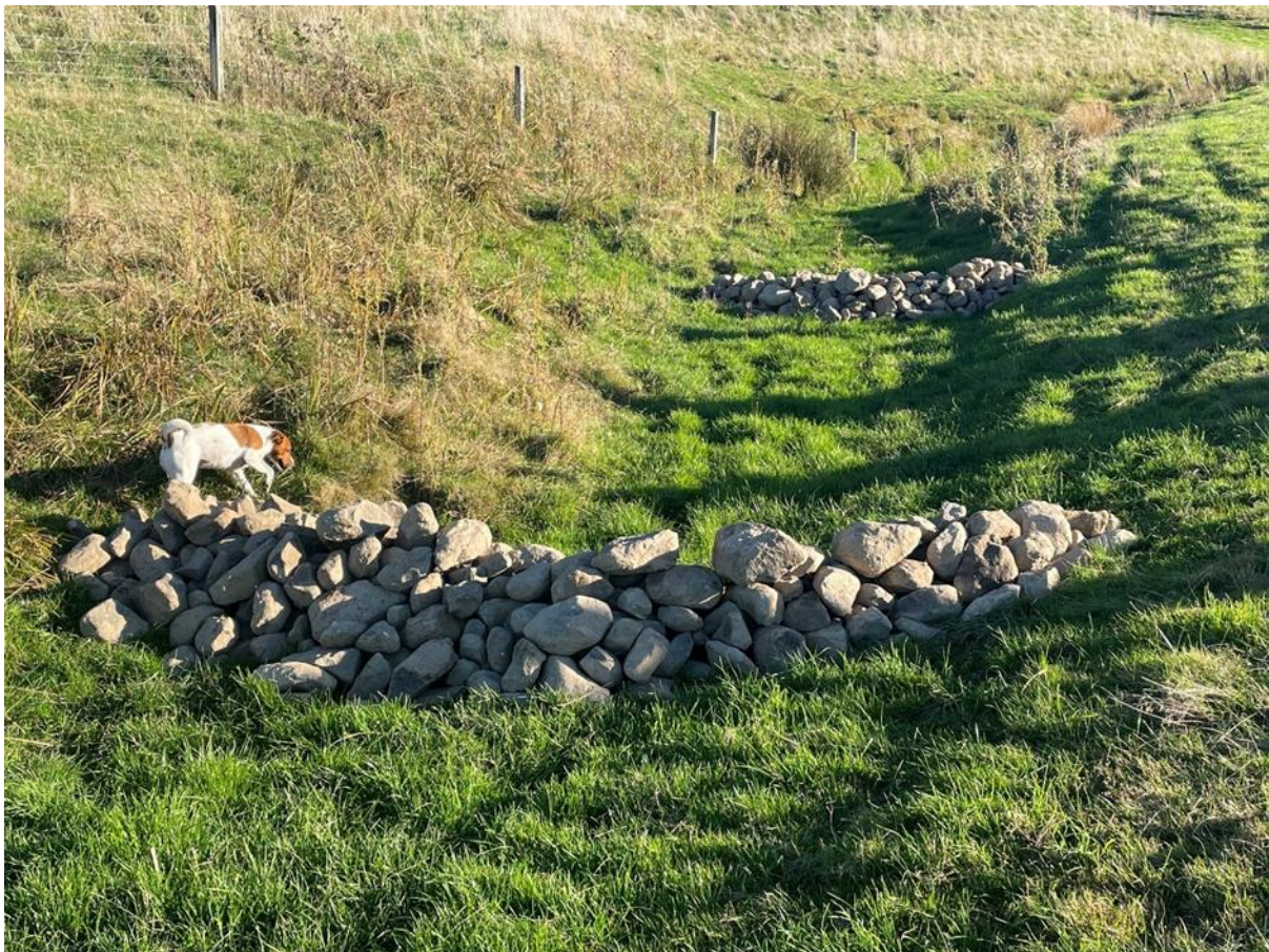
Figure 20. Daisy chain (there are three of these structures in a row, one is hidden from view) of boulder check dams within an ephemeral (overland flow) pathway on a Southland farm – Jack Russel for scale (courtesy of Chris and Andrea Bullied, Waimea Catchment Group).
