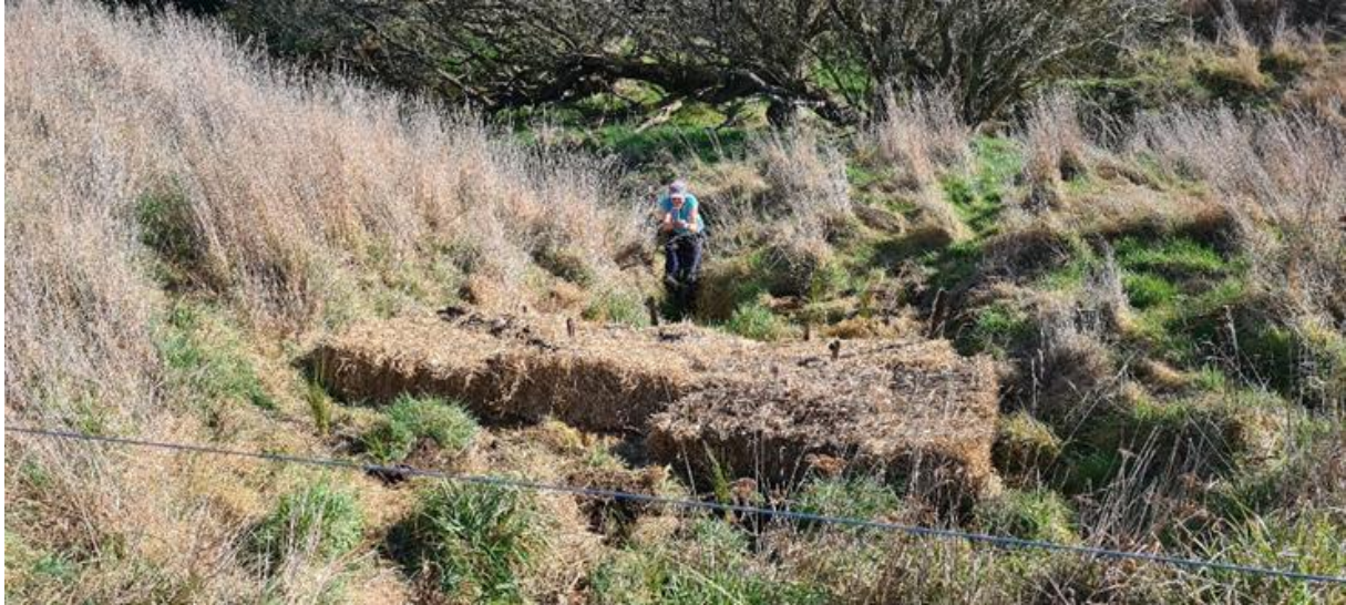
Figure 9. Staked haybales within an ephemeral flowpath that is connected to a perennial stream (Thriving Southland).
