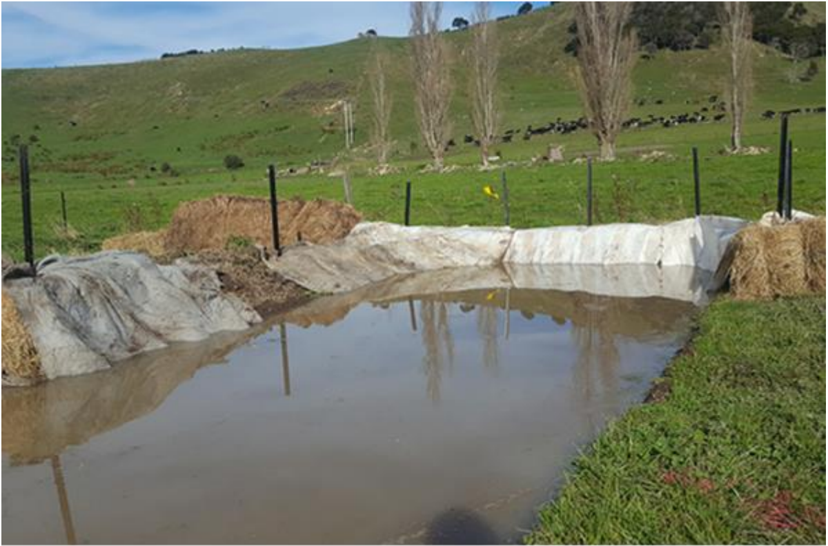
Figure 16. A sediment retention structure (sump) at the end of a runoff pathway, before an open drain (Aqualinc). The open drain is behind the end of the retention sump. The water gradually infiltrates through the soil to the stream, leaving the sediment behind.
