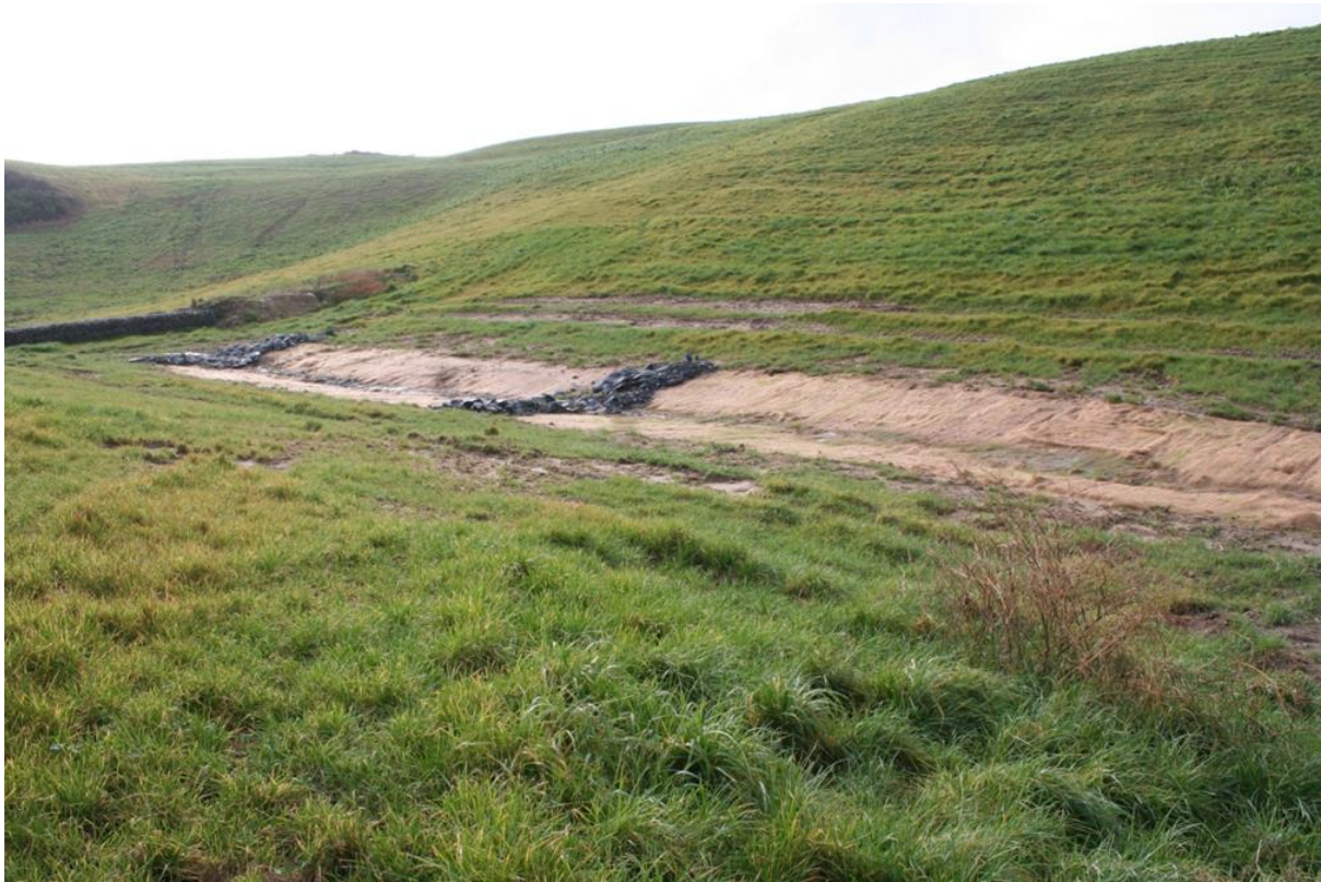
Figure 18. A recently installed interception (detention) swale at the base of a steep hillslope (Tonkin & Taylor). Note the rock and earth wall in the top left and the use of geotextile and rock battering along the ephemeral flow path. This is an example of daisy chaining. Over time the area will be colonised by plants.
